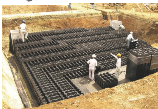
▼ Installation of Cross-Wave
