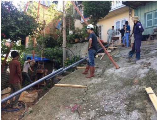
Emergency Survey and Installation of Monitoring Post for Prevention of Landslides
