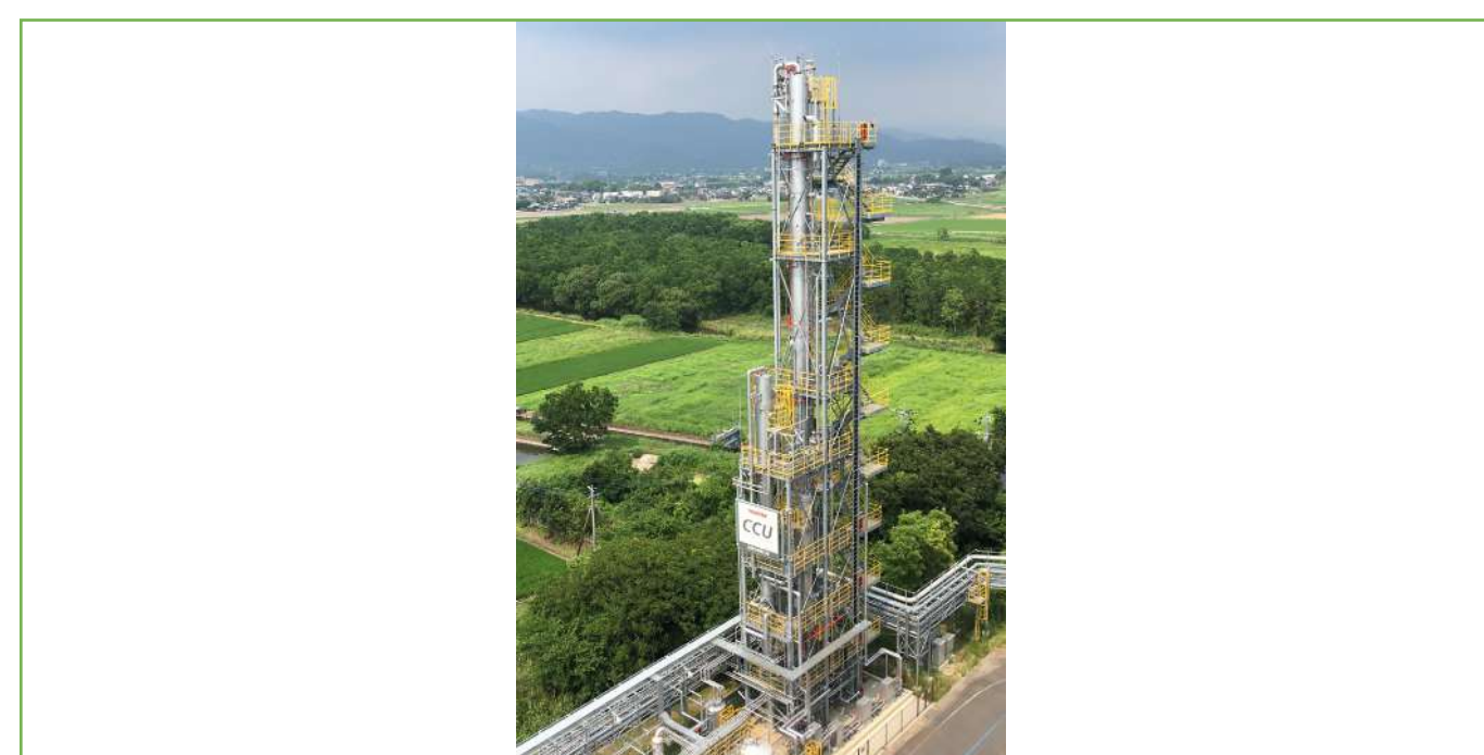
図1 佐賀市清掃工場様向けCO 2 分離回収商用設備 Fig.1 The world's first commercial CCU plant for waste incineration plant in Saga city
