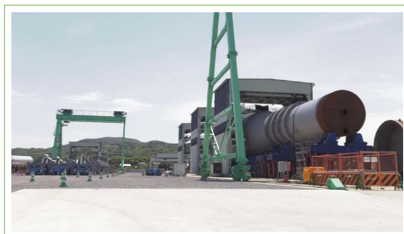
上部鋼製部製造 Manufacturing of upper steel part
