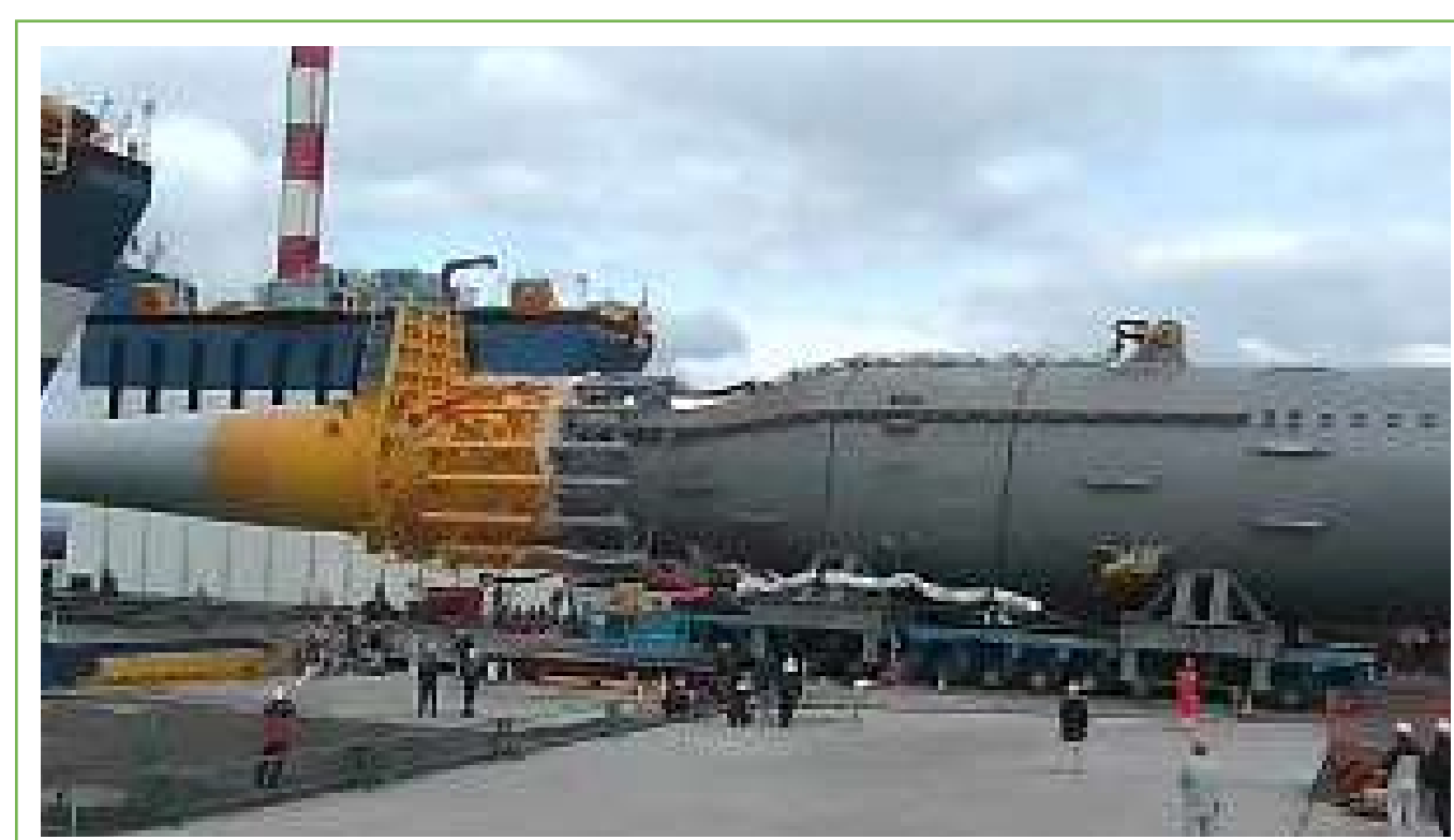
浮体の半潜水船への積み込み Loading the floater onto the semisubmersible vessel
