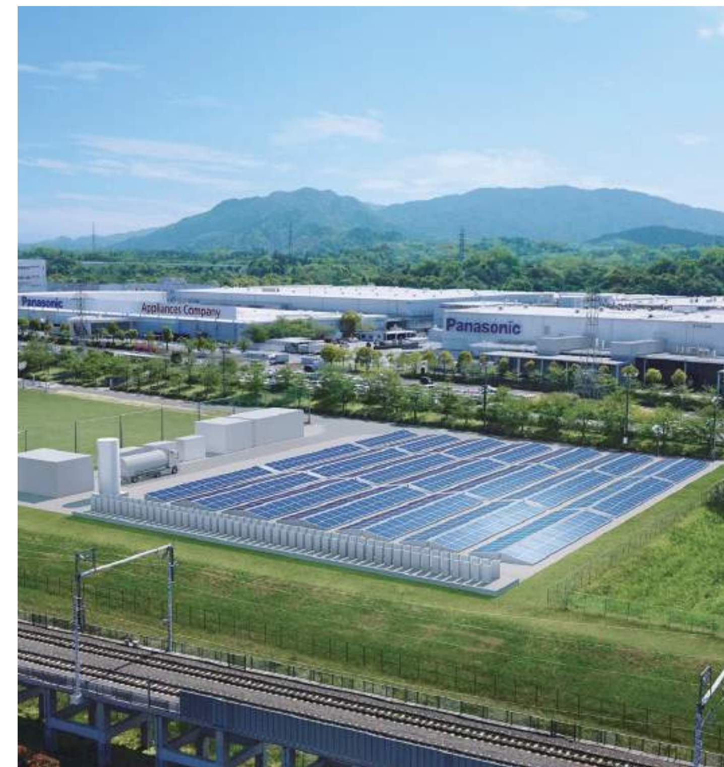
RE100 工場 First hydrogen-based plant using only renewable(RE100 solution)
