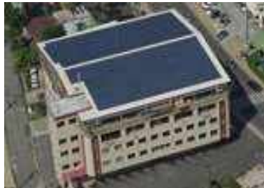
Installing solar PV system, PCKK, Palau Maldives
