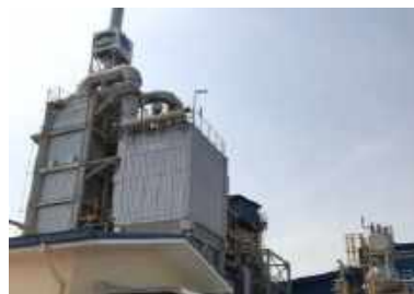
Waste to Energy Plant, JFE engineering, Myanmar
