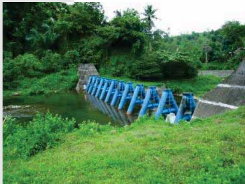
Slit dam for debris flow (Philippines)
