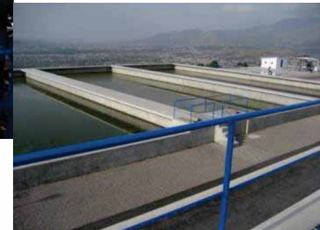
Water supply facility (Pakistan)
