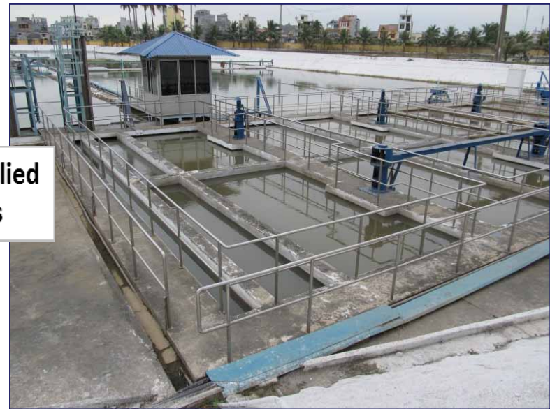
Main water treatment plant (An Duong Water Treatment Plant)
