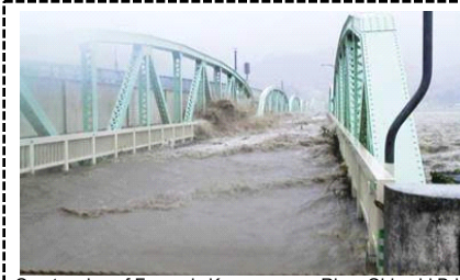
Overtopping of Formerly Kumanogawa River Ohhashi Bridge (photo taken from the right bank)
