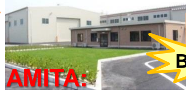
AMITA: Waste treatment operator
